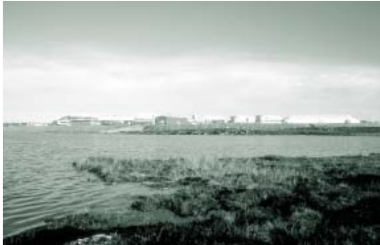
View of Ekati™ main camp complex across Kodiak Lake BHP BILLITON DIAMONDS INC.
