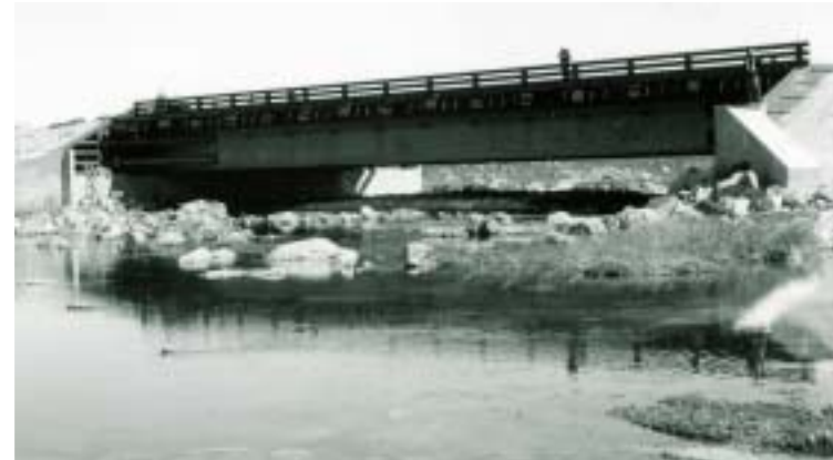
Fox Bridge crossing the Nero-Nema stream AGENCY
