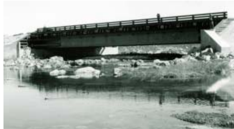
Fox Bridge crossing the Nero-Nema stream AGENCY
