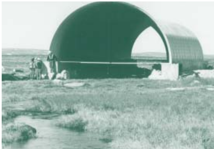
Culvert on Sable Haul road at Pigeon stream crossing AGENCY
