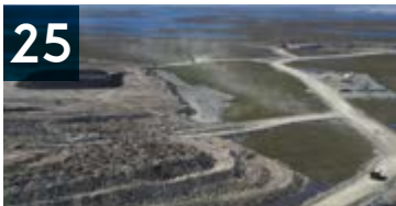
25 JAY EXPANSION PROJECT
