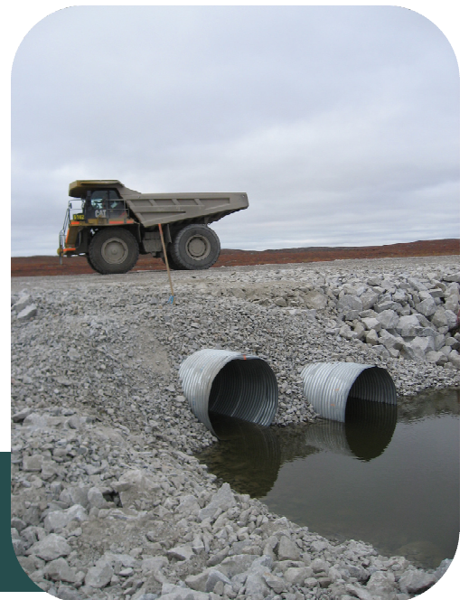
Photo from the Jay North Road. Also depicting culvert B-06.
