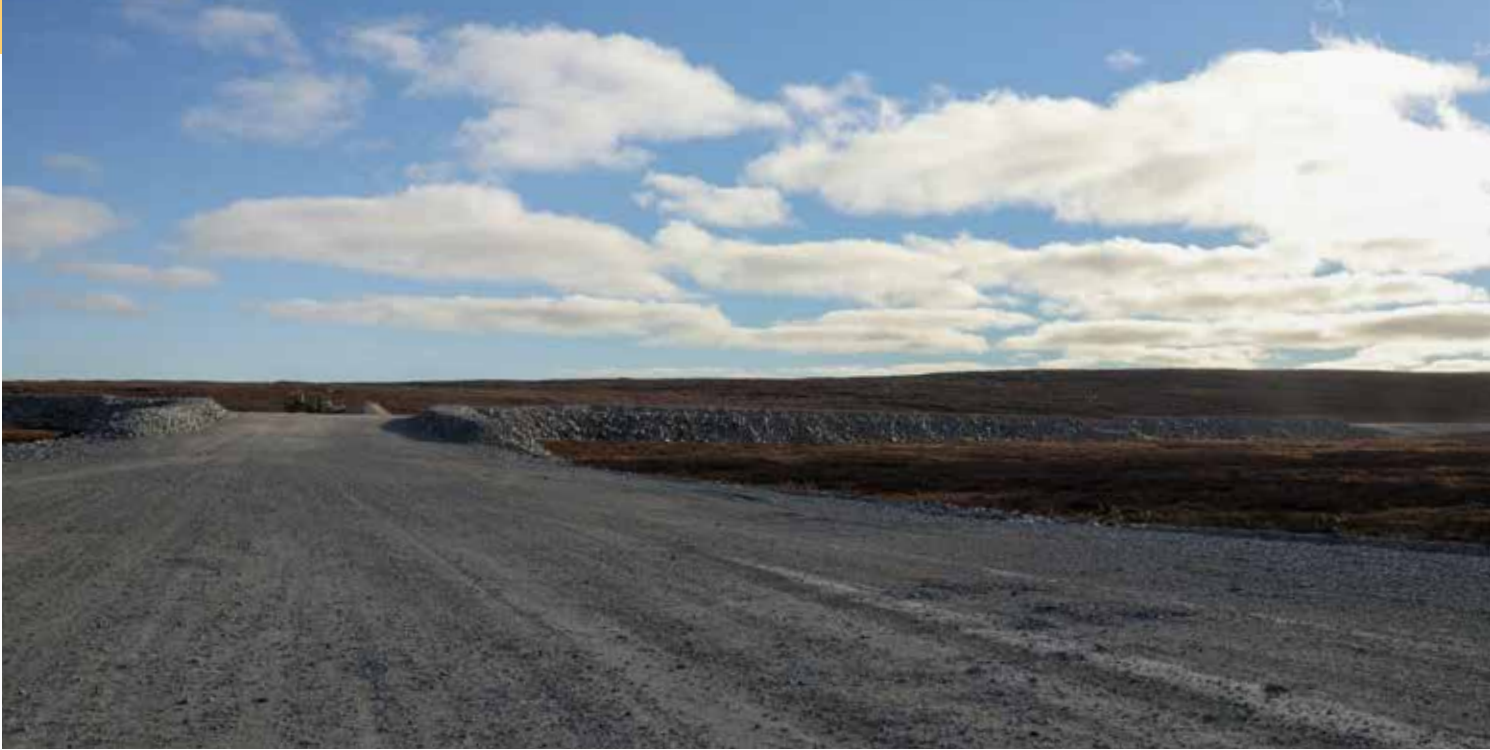
Berms along the Lac du Sauvage Road - 2022 site visit
