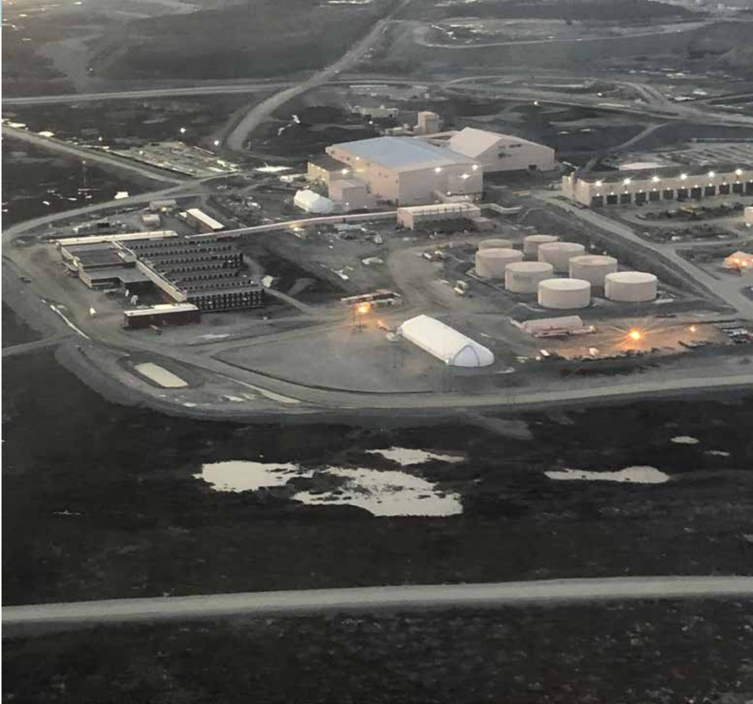
Main camp with accommodations, process plant, main tank farm, and workshops
