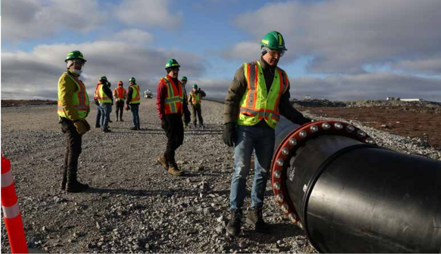
Directors observing Point Lake discharge pipe - 2022 site visit
