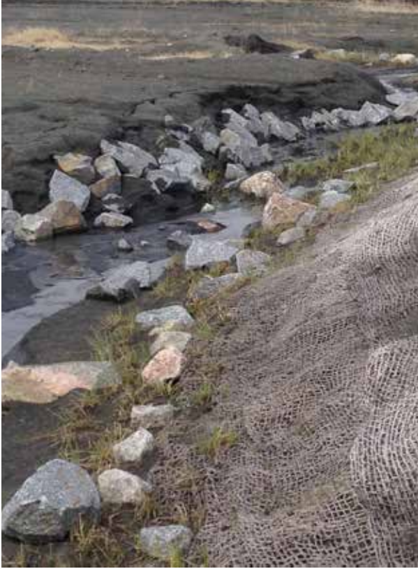
Revegetation webbing on the LLCF - 2016 site visit
