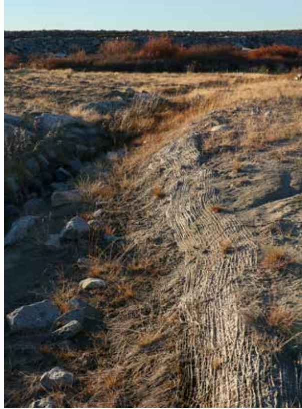
Revegetation webbing on the LLCF - 2022 site visit
