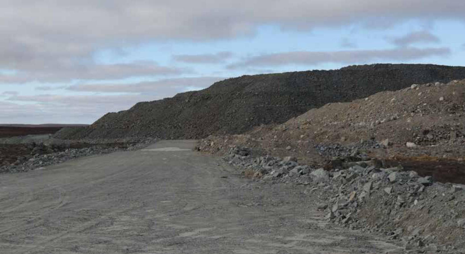
Wasterock pile in the back and overburden stockpile in the front - 2022 site visit
