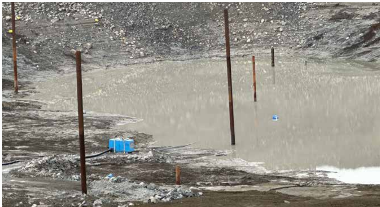
Point Lake pit dewatering October 2024.
