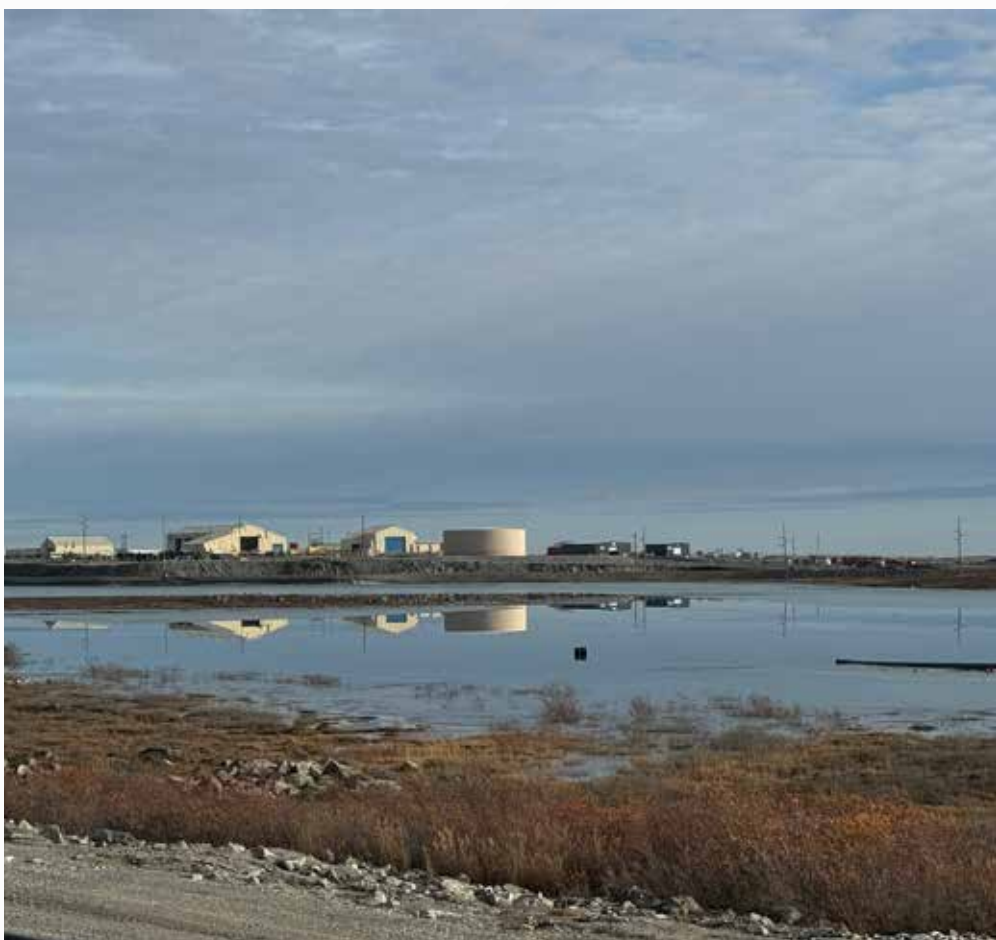
King Pond Settling Facility and Misery Camp in background 2024.
