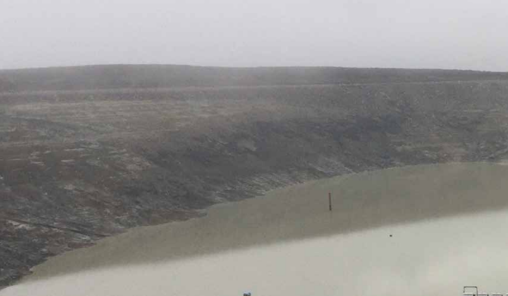
Point Lake during the dewatering phase, 2023.
