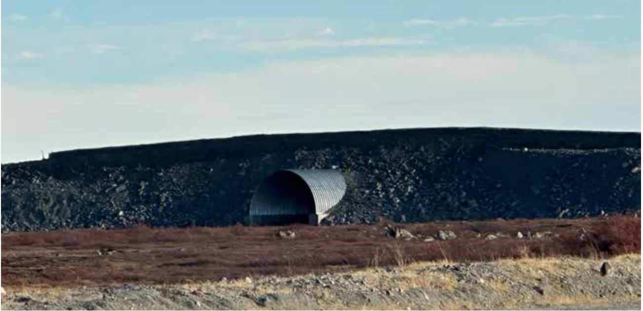
Culvert under Sable road, 2024.
