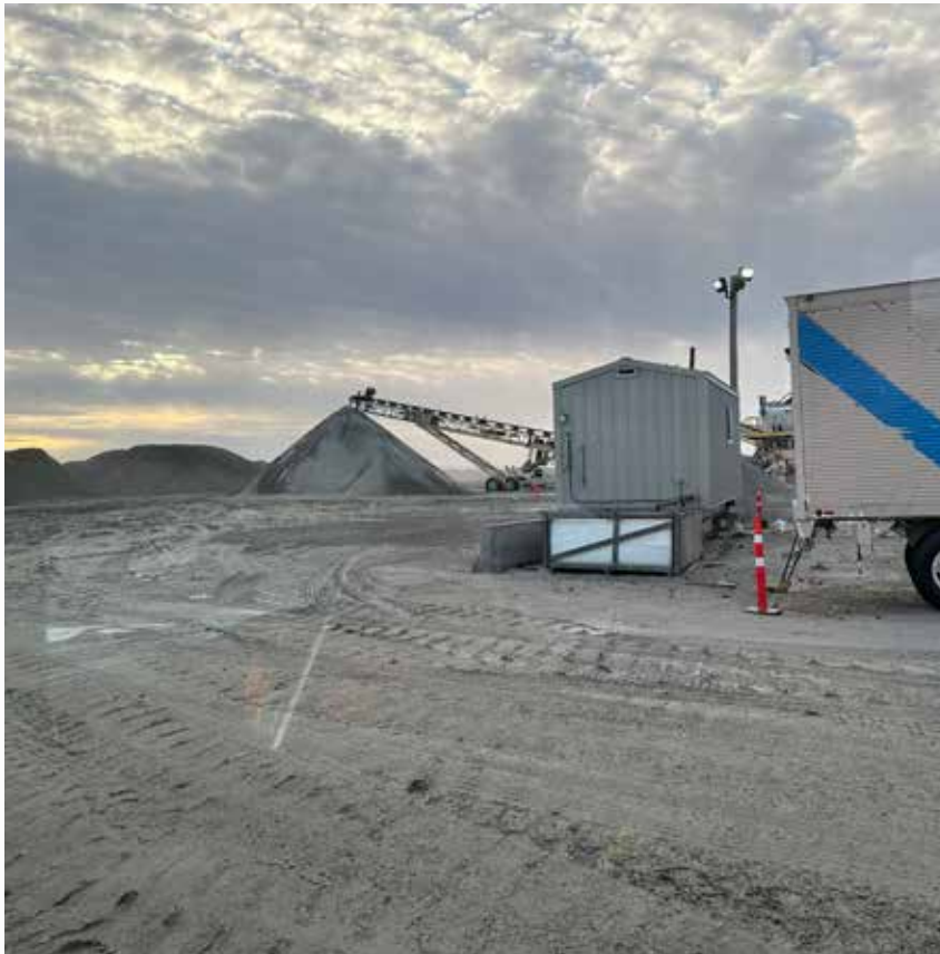
Sable crusher pad 2024.
