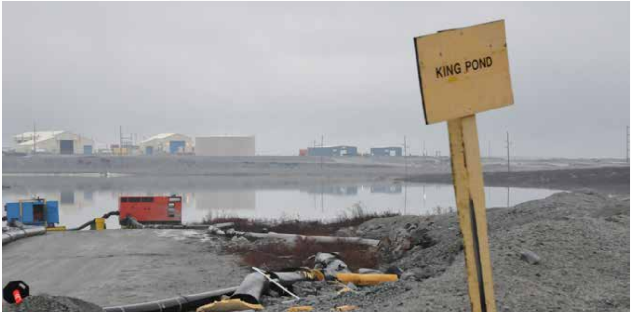
King Pond Settling Facility during mine site visit 2023.
