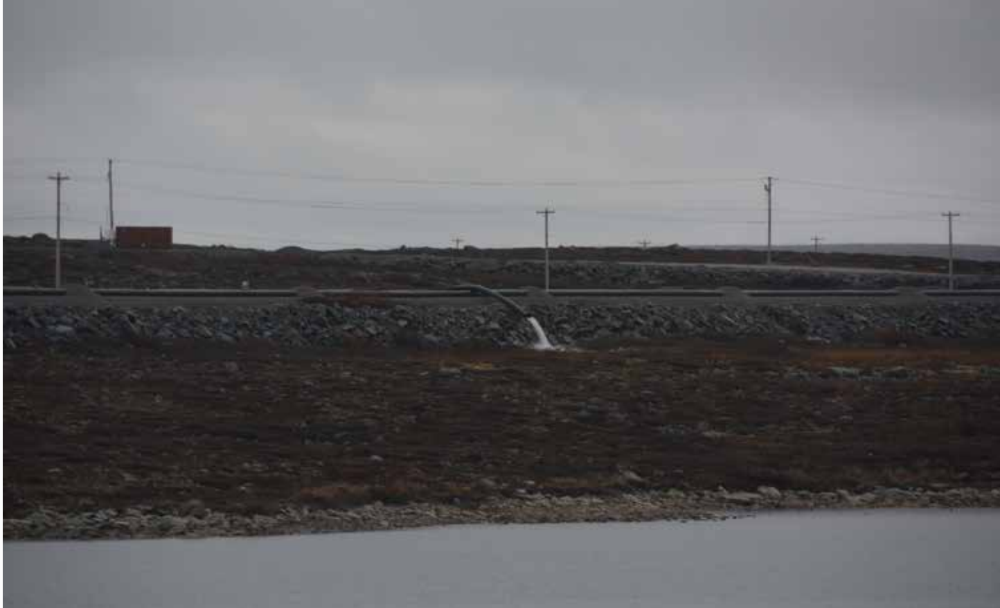
Minewater discharge into Cell D of LLCF taken during site visit 2023.
