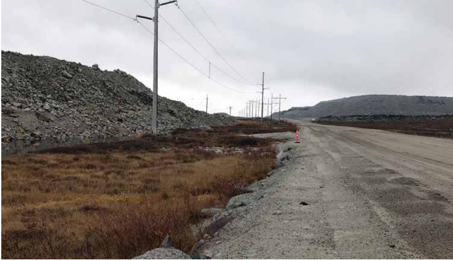
Misery Road with Lynx crusher pad on the left and Lynx/Misery Waste Rock piles on right taken during site visit 2023.
