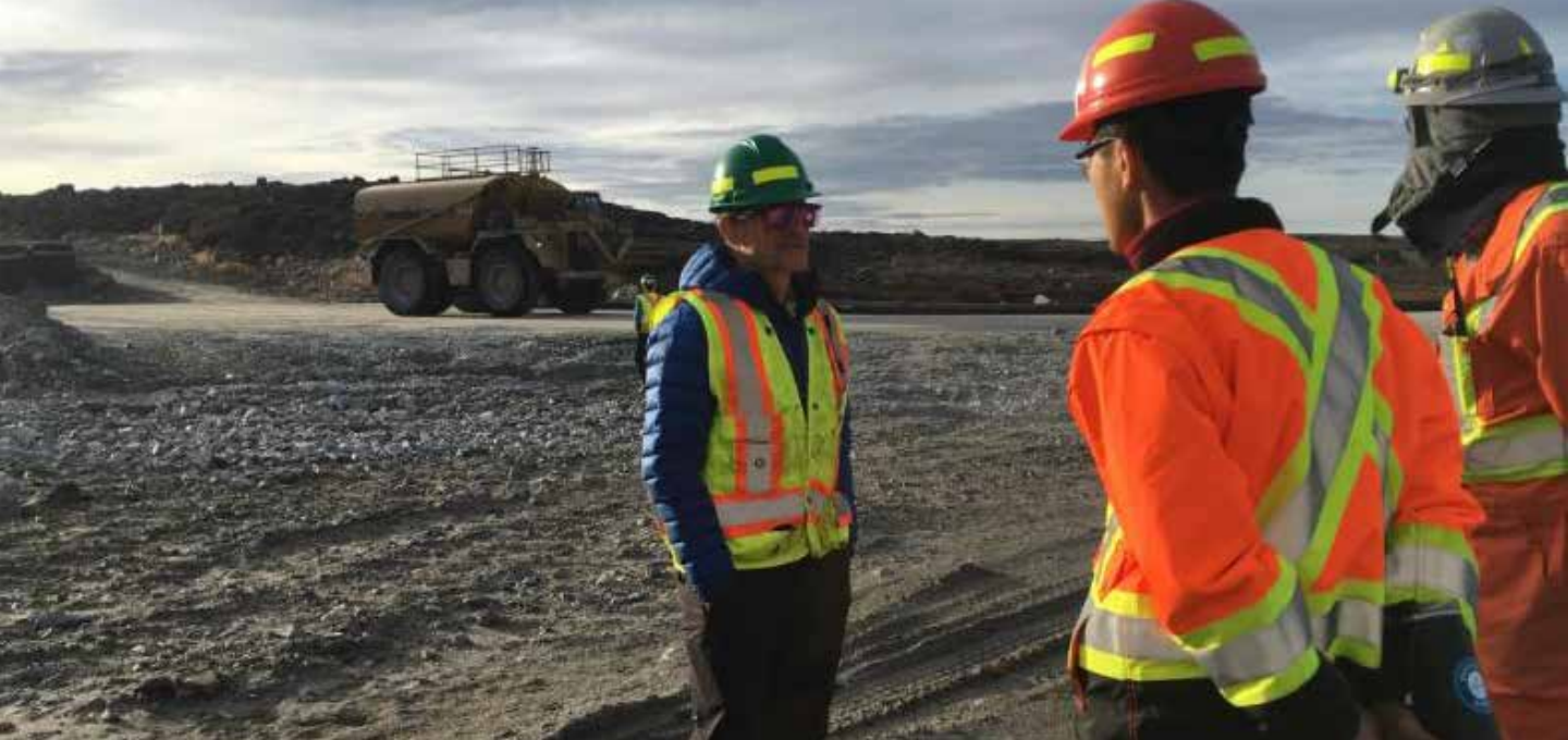
King Pond dam 2024.
