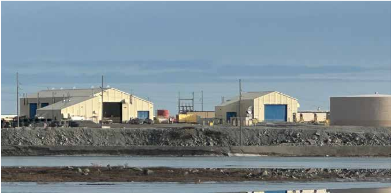
Misery camp and King Pond Settling Facility.
