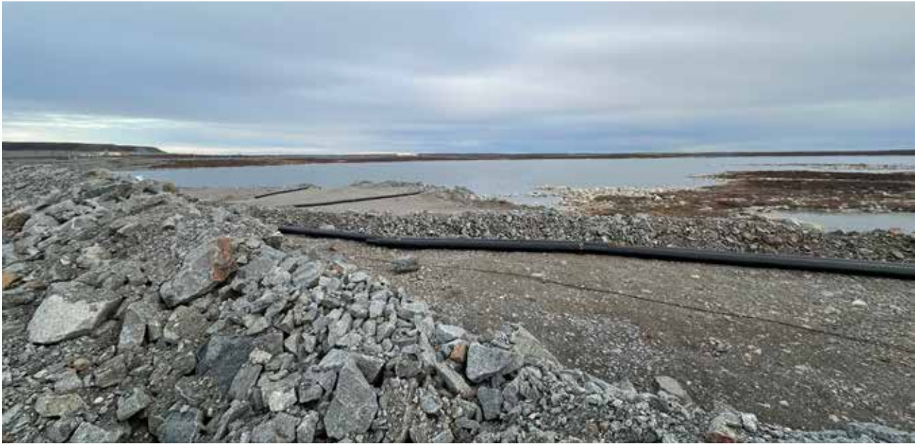
Cell D of the Long Lake Containment Facility.
