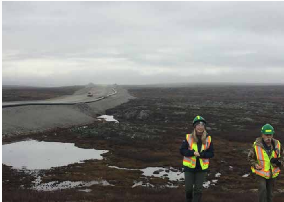
Typical section of road with insulated water pipe at Ekati Diamond Mine 2023.
