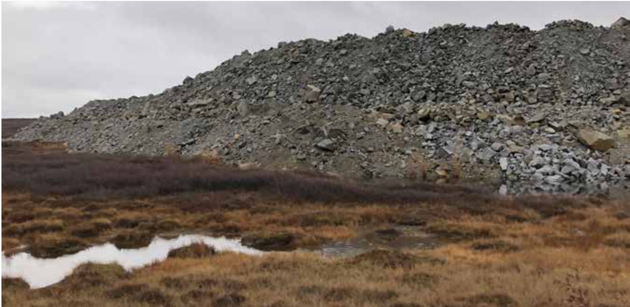
Lynx crusher pad and adjacent wetland taken during site visit.
