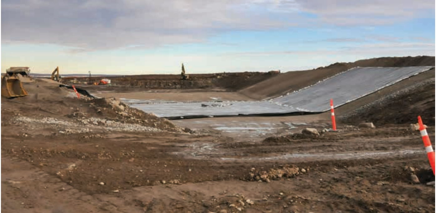
Construction of the Point Lake seepage collection channel, October 2024
