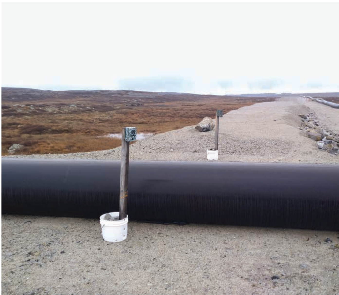
Wildlife cameras beside a dewatering pipeline during the Point Lake dewatering
