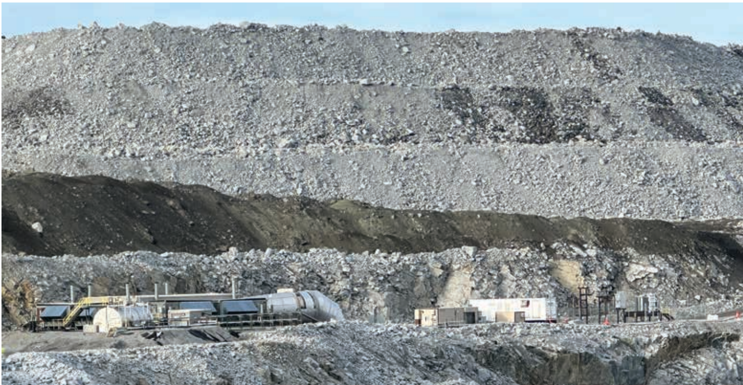
Misery underground infrastructure, October 2024
