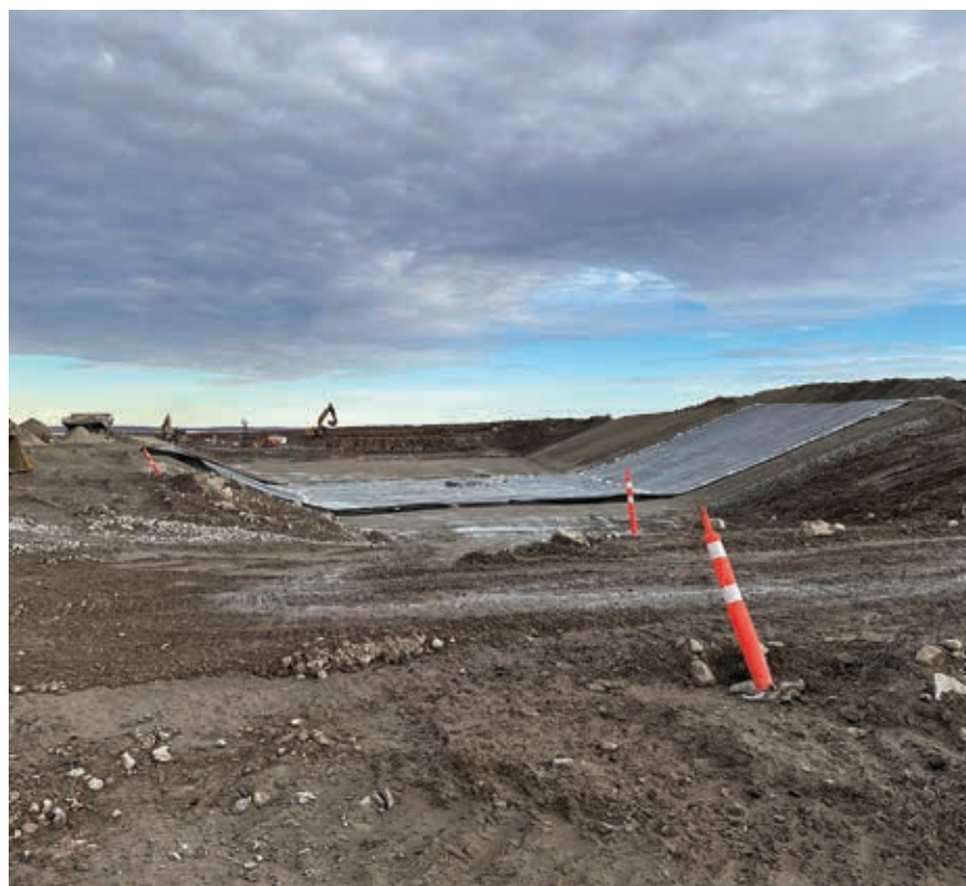
Construction of the Point Lake seepage collection ditch, October 2024
