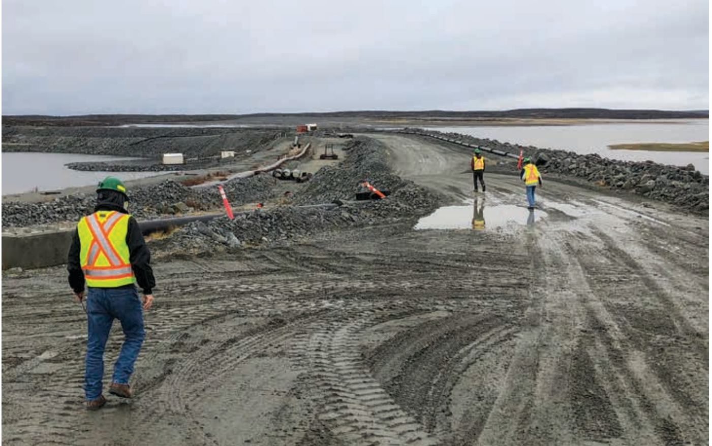
Directors walking along Dike B of the Long Lake Containment Facility, October 2023
