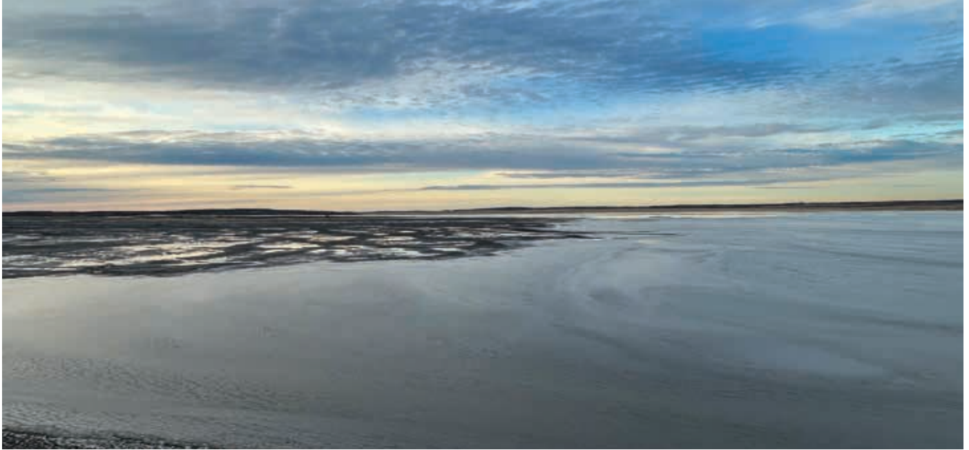
Cell C of the Long Lake Containment Facility, October 2024
