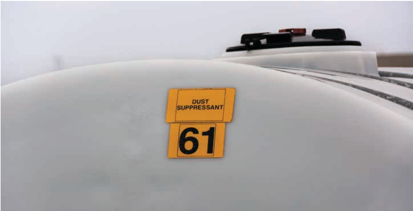
Dust suppressant stored in container on site
