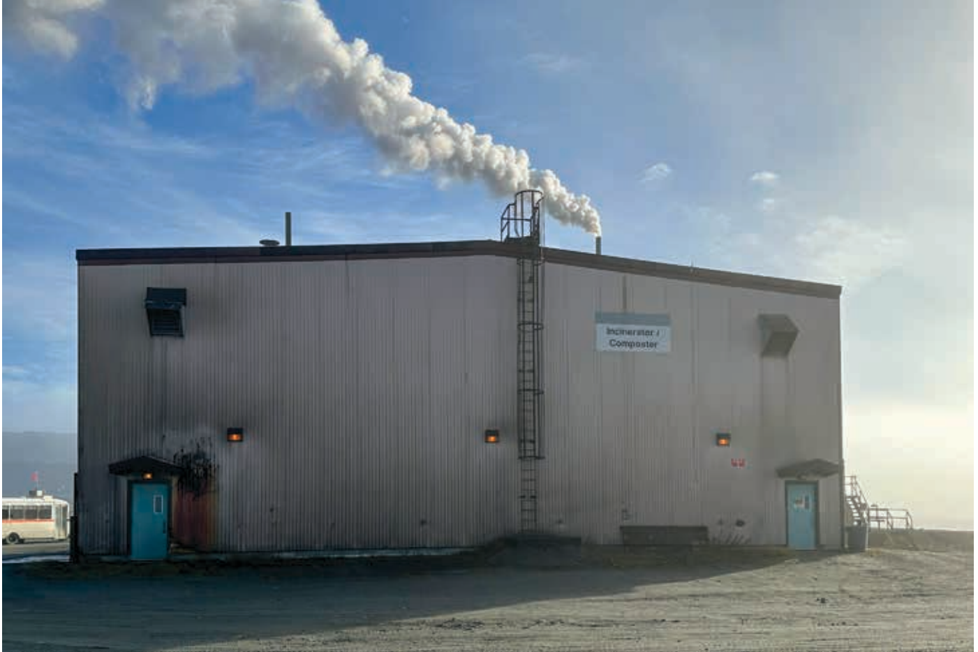
Solid waste incinerator building
