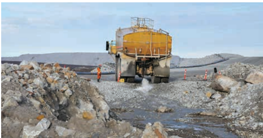
Wastewater transferred by truck from the Point Lake seepage collection channel to King Pond
