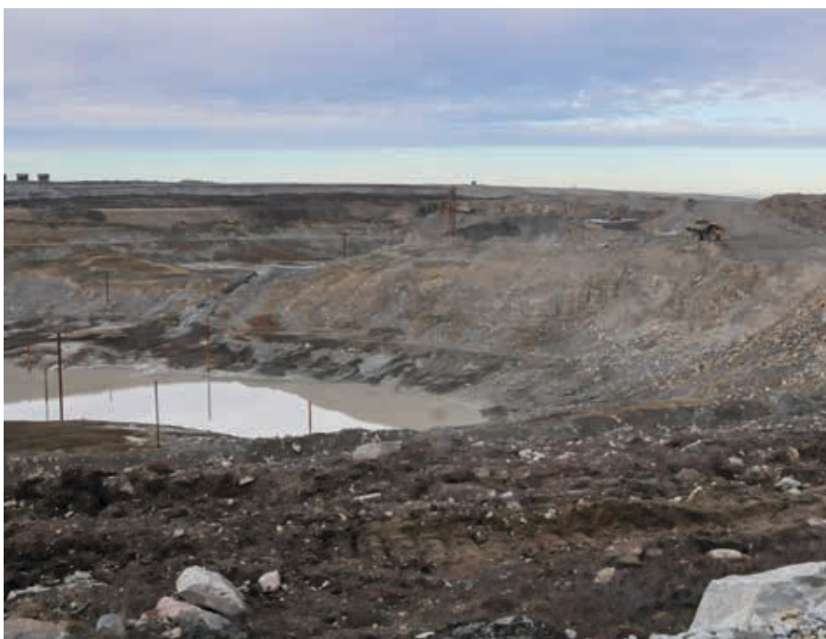
Initial stripping of Point Lake, October 2024
