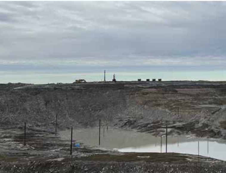
Point Lake pit at the start of construction, 2024
