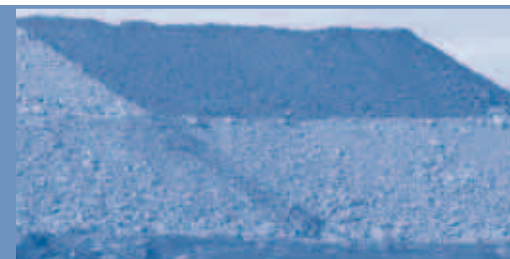
Coarse kimberlite reject storage area within the waste rock pile. AGENCY
