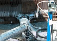
Protection on pipes installed to prevent wolverine access
