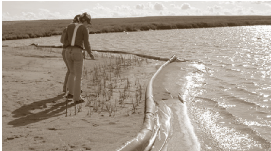
Shoreline erosion protection at Ekati
