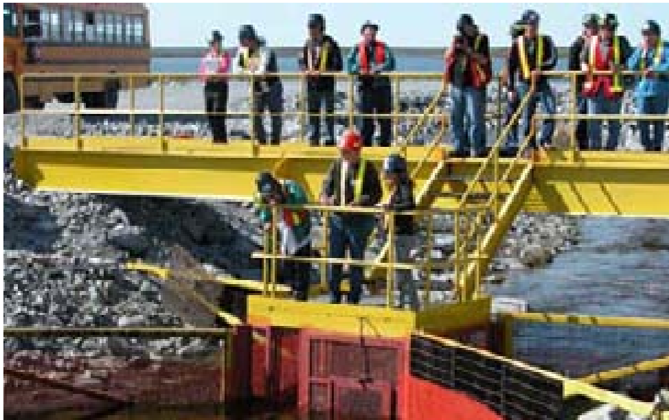
Ekati visitors tour the Panda Diversion Channel fish box
