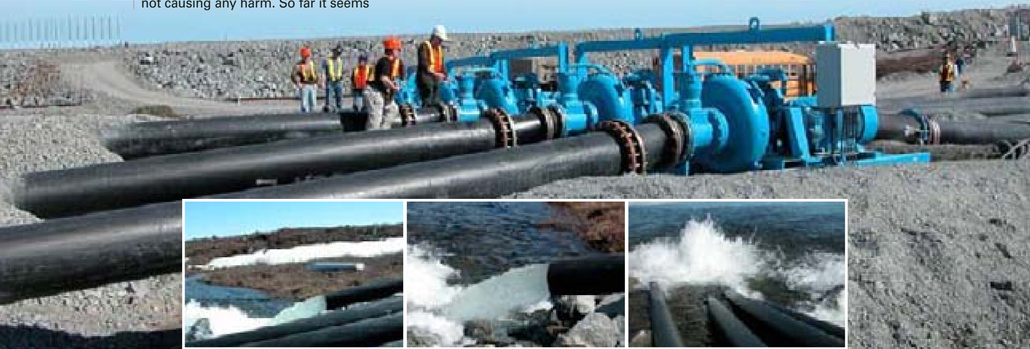
Pumping water from Long Lake into Leslie Lake
