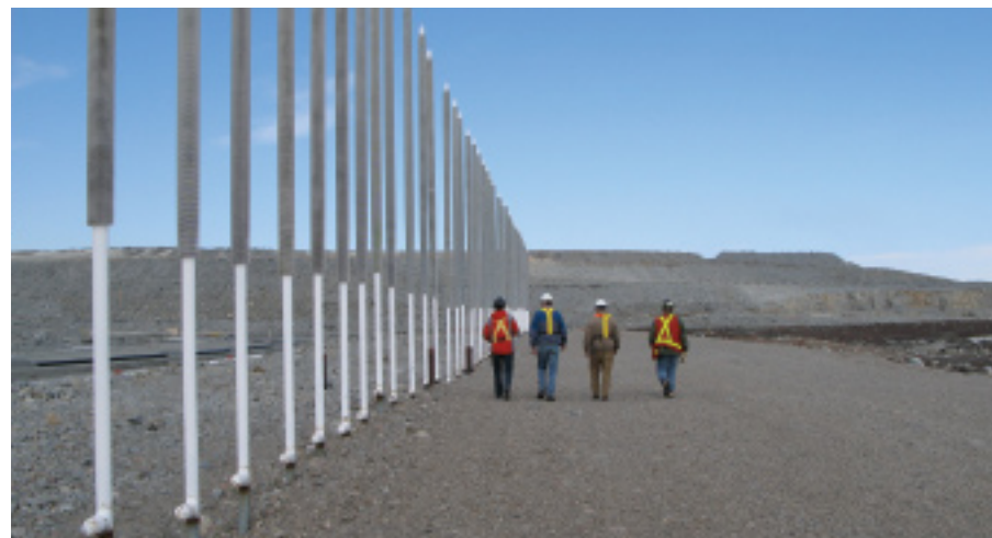
Thermosyphons at Upper Panda Dam.
