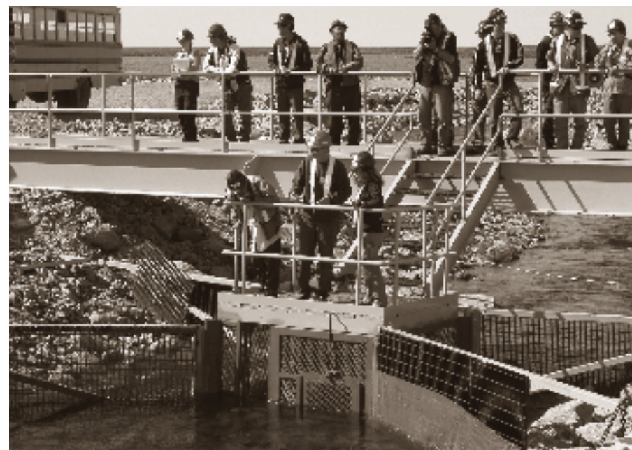
Fish box in the Panda Diversion Channel.
