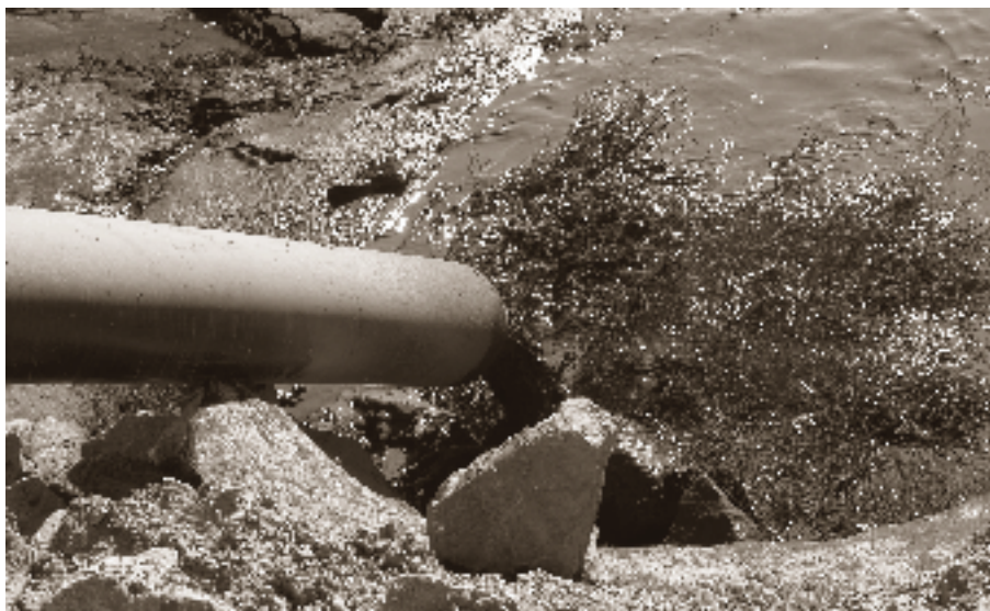
Tailings discharge point at cell A of the Long Lake Containment Facility.
