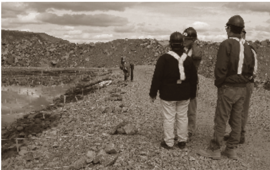
Flagging tape on lines across the contaminated snow containment facility.
