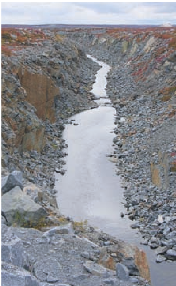
Panda Diversion Channel.
