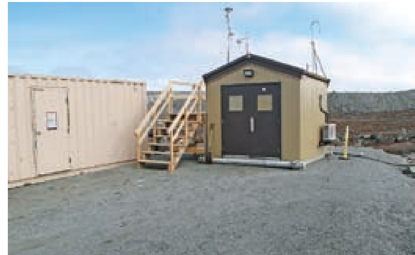
Continuous air quality monitoring building (new location).
