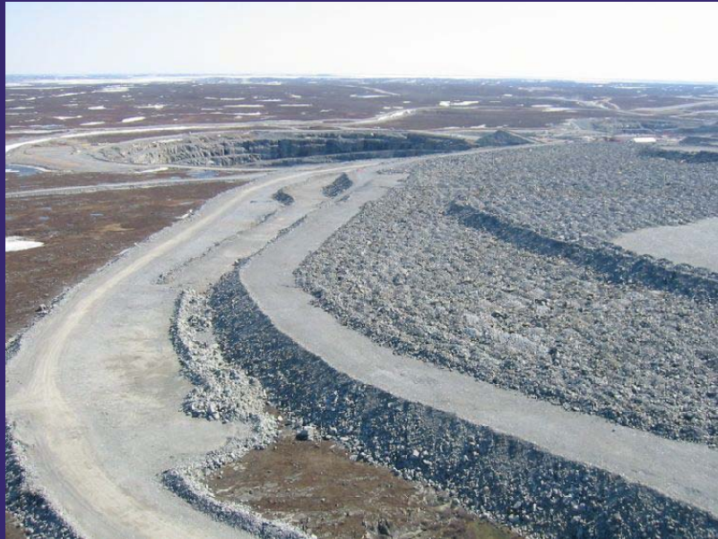
Main waste rock pile, Panda Pit in Background
