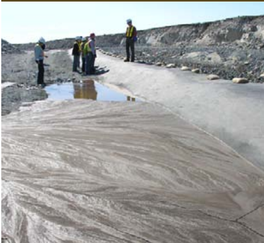
Bench on newly-widened PDC to capture sediments, June 2011.
