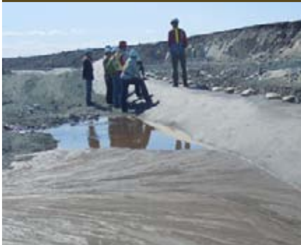
Sediment capture on widened part of Panda Diversion Channel.
