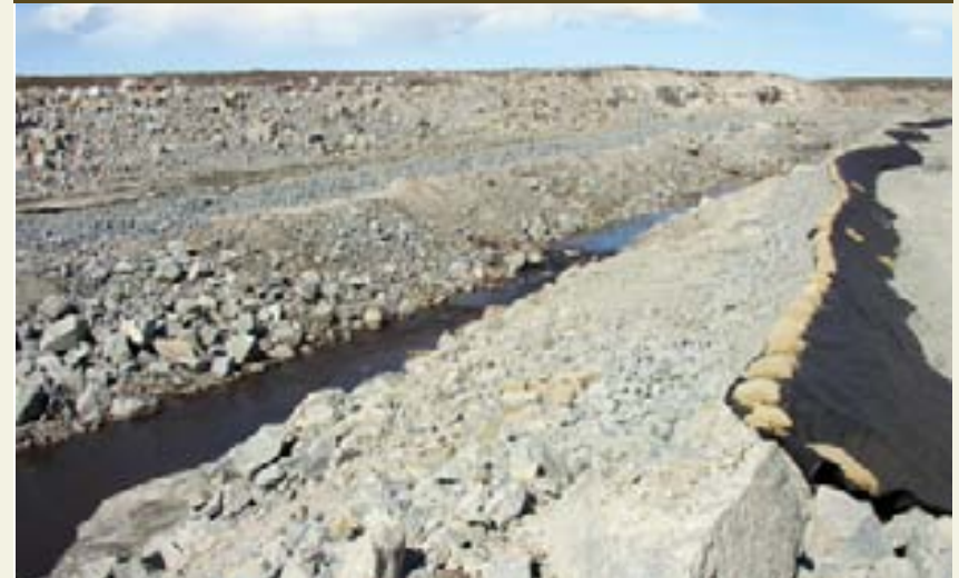
Widened part of Panda Diversion Channel, June 2011.
