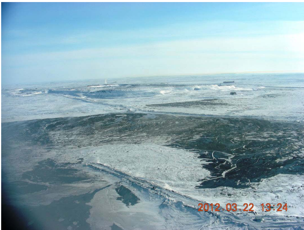
Cell B new jetty – It appears Cell B is nearing its maximum hold capacity. Only a small area of exposed tundra remains uncovered in Cell B.
