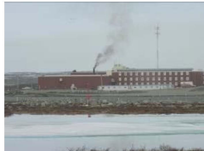
Current Incinerator in Operation
