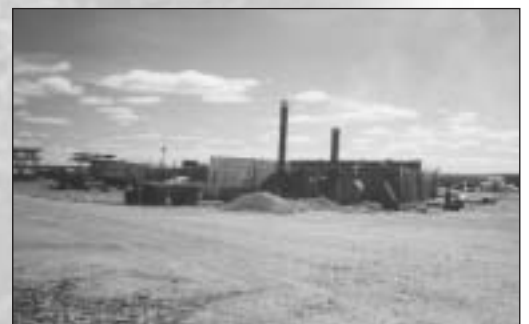
Waste Incinerator at the Misery Camp Photo: Agency
