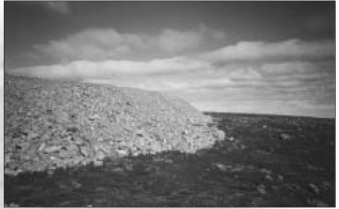
Toe Berm on the Panda Waste Rock Pile Photo: Agency
