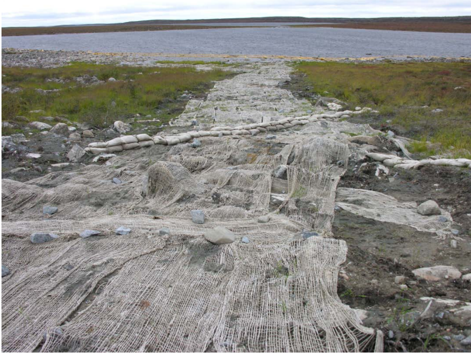
Burlap and sand bags to prevent erosion
