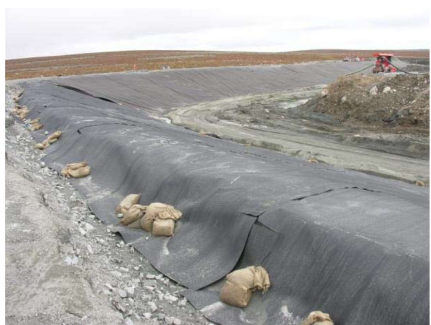
Liner and berm being built at north end of Cell B
