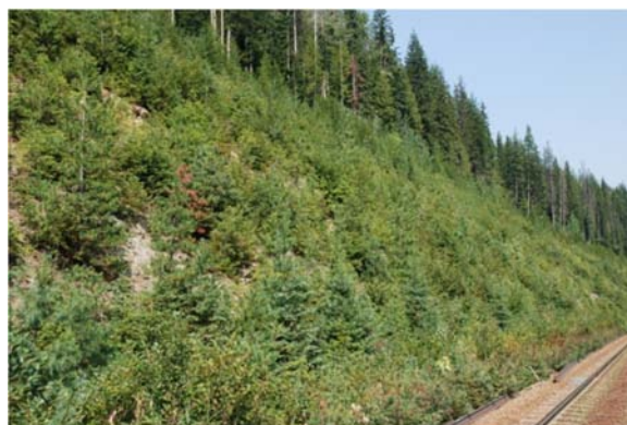
Photographs 3 (left) and 4 (right). Seeding Sitka Alder on this 0.8:1 rock cut in October, 1986 (left) resulted in re-establishing the natural successional processes that by August, 2009 resulted in a cover of healthy conifers on the rock cut.
