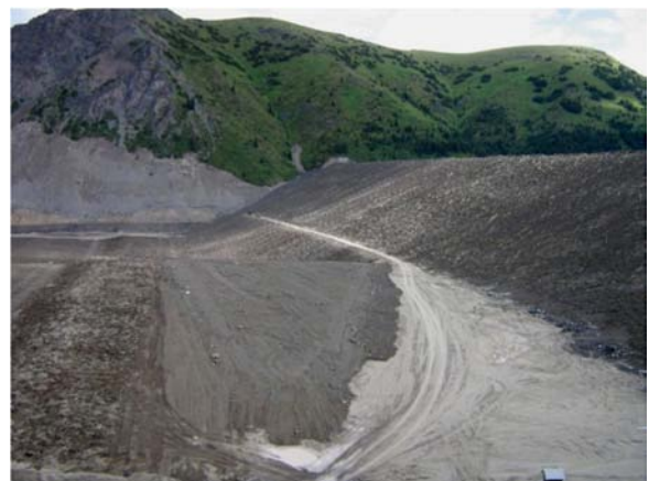
Photographs 8 (left) and 9 (right). Rough and loose terrain traps winter snow (left) and prevents erosion on steep slopes (right) by preventing water from running down the slope.
