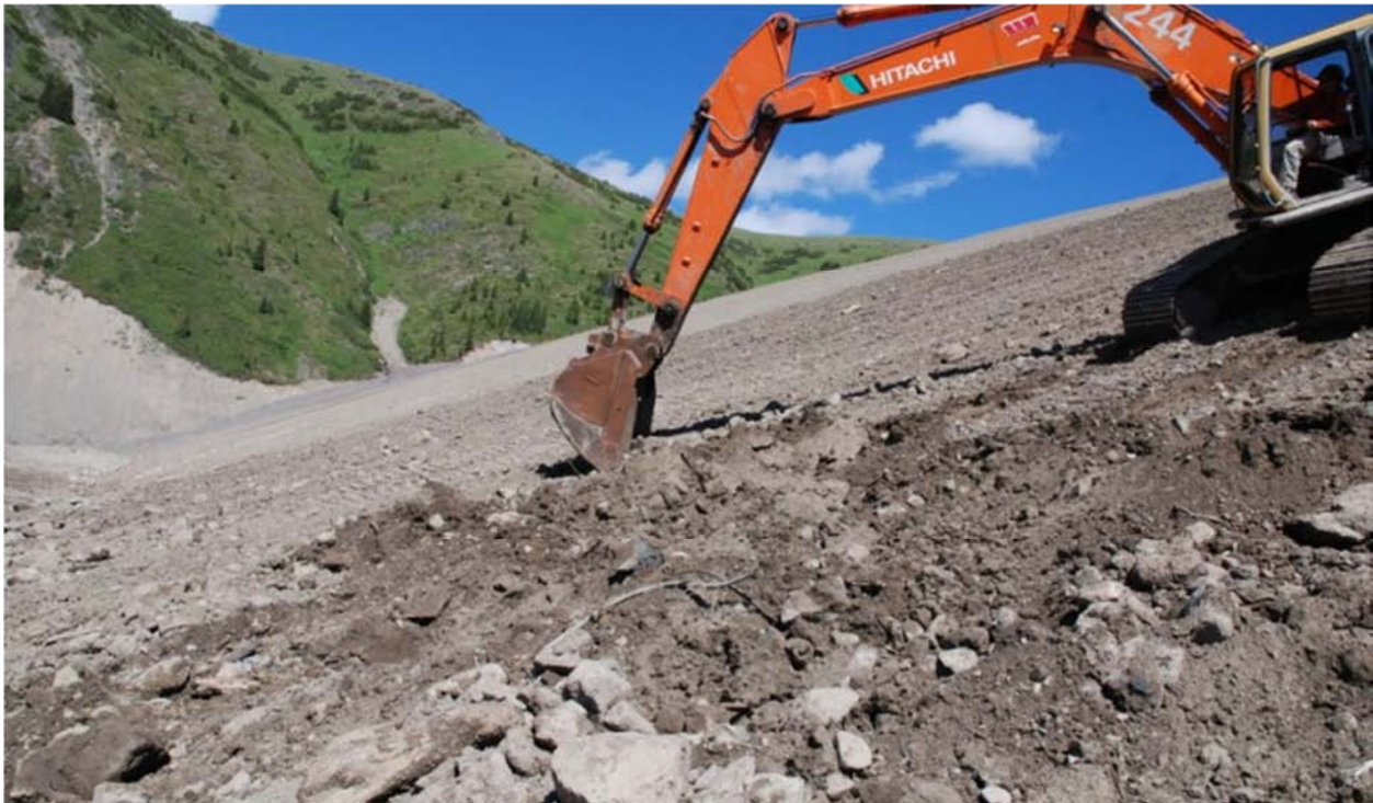
Photograph 10. Rough and loose surface configurations are easy to construct using a large excavator and cost about one-third the cost of traditional hydroseeding.
